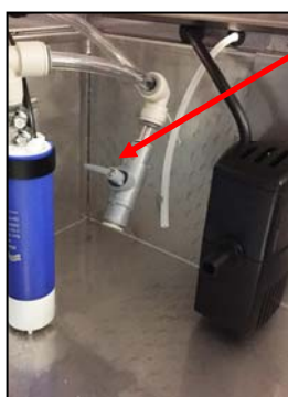
Fig. 3 Priming valve in OPEN position
