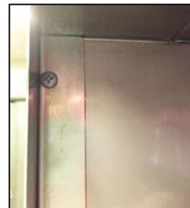
Fig 6. Screws for air returns
